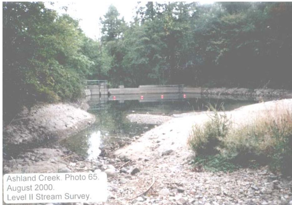
Figure IX-14: Fine sediment and coarse granitic sand stored in Granite Reservoir. Photo by Siskiyou Research Group, September 1999 (SRG 2001).
