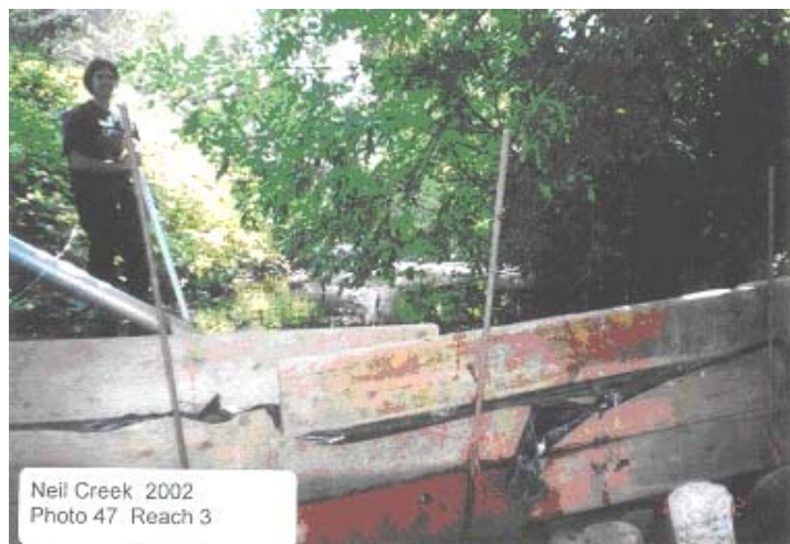
Figure IX-33: Irrigation diversion structure made out of boards, rocks, and plastic in lower Neil Creek along Hwy. 66. Photo: Siskiyou Research Group, September 2001 (SRG 2002a).
