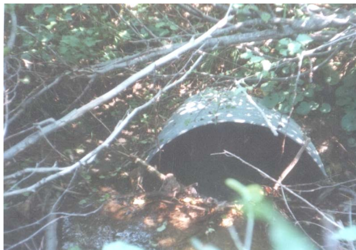
Figure IX-36: Neil Creek culvert blocked by granitic sand and debris, far upstream in T40s-R1e-Sec. 23. Photo: Ecosystems Northwest, September 1999 (ENW 2000).
