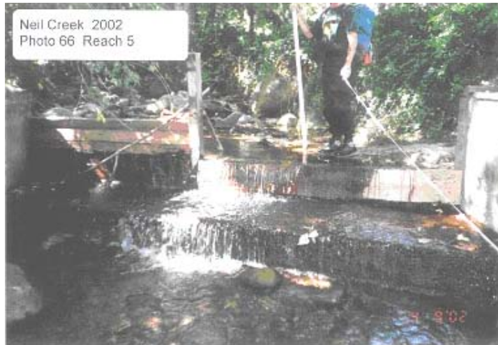
Figure IX-31: Concrete irrigation diversion in Neil Creek. Photo: Siskiyou Research Group, Sept. 2001 (SRG 2002a).
