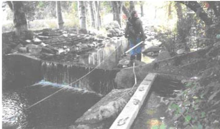
Figure IX-32: Three-foot high irrigation diversion structure on Ashland Creek just upstream of Nevada Street. Photo: Siskiyou Research Group, August 2000 (SRG 2001).
