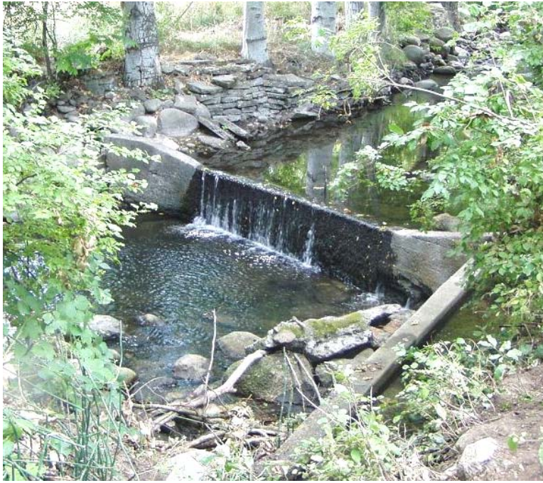
Figure XII-6: Fish barrier on Ashland Creek at Smith/Meyer/Roper diversion, August 2007.
