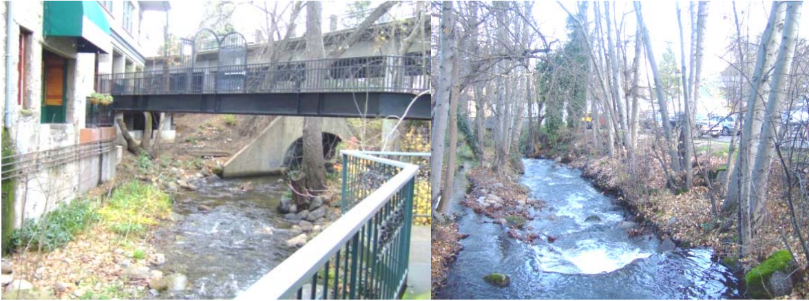
Figure IX-11: Ashland Creek through the urban corridor. Left: Ashland Creek flows between buildings on its left and right and is forced through the Lithia Way culvert (background) by road fill. The Lithia Way culvert did not contain all the flood water in the 1997 flood. Right: Looking downstream from the walking bridge next to the Lithia Way culvert. The white area in the lower center of the photo shows where the stream drops over a diversion dam (and partial fish migration barrier) shunting water into the Helman ditch, in the left of the photo. There is only a single line of trees on both sides of the stream through this section. A parking lot next to Water Street is immediately adjacent to the narrow riparian area. During the floods of 1974 and 1997, this lot and Water Street itself were flooded. Photos © Jeannine Rossa, December 2007.
