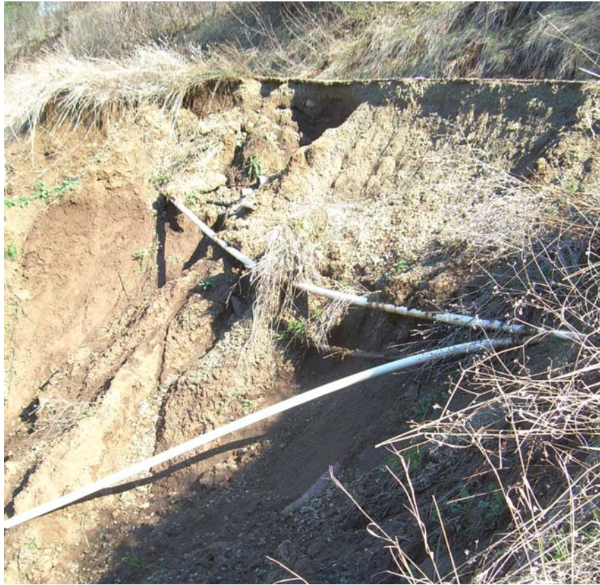
Figure XII-5: Failing road prism in Sec. 31, 38-1East (above Butler Ford).
