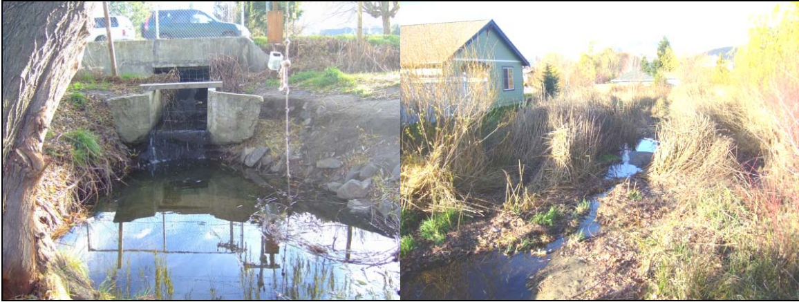
Figure IX-26: Roca Creek, downstream of East Main Street. Left: Roca Creek exits an underground pipe below East Main. Right: After exiting the pipe, the stream flows through a constructed wetland filled with cattails and other wetland vegetation. The wetland filters and cleans the stream water and also traps a large amount of granitic sand and fine silts; residents are concerned that the stream may damage their properties. Photos © Jeannine Rossa, December 2007.
