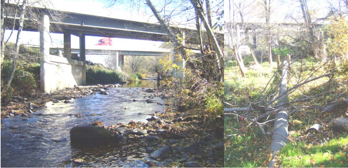
Figure IX-28: Left: Bear Creek looking upstream underneath the Interstate-5 bridges. A large, vegetated berm is visible behind the bridge abutment in the left of the photograph. Right: Part of the sewer pipe system for the City of Ashland. Most of the sewer pipe is underground. The Interstate-5 bridge over Bear Creek is visible in the background. Photos © Jeannine Rossa, November 2007.
